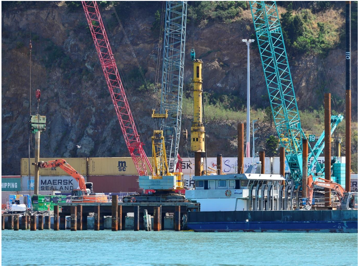
Figure 3.1. Construction works at Cashin Quay 2, Lyttelton. The BSP hammer in the centre and a pile being positioned on the left.
