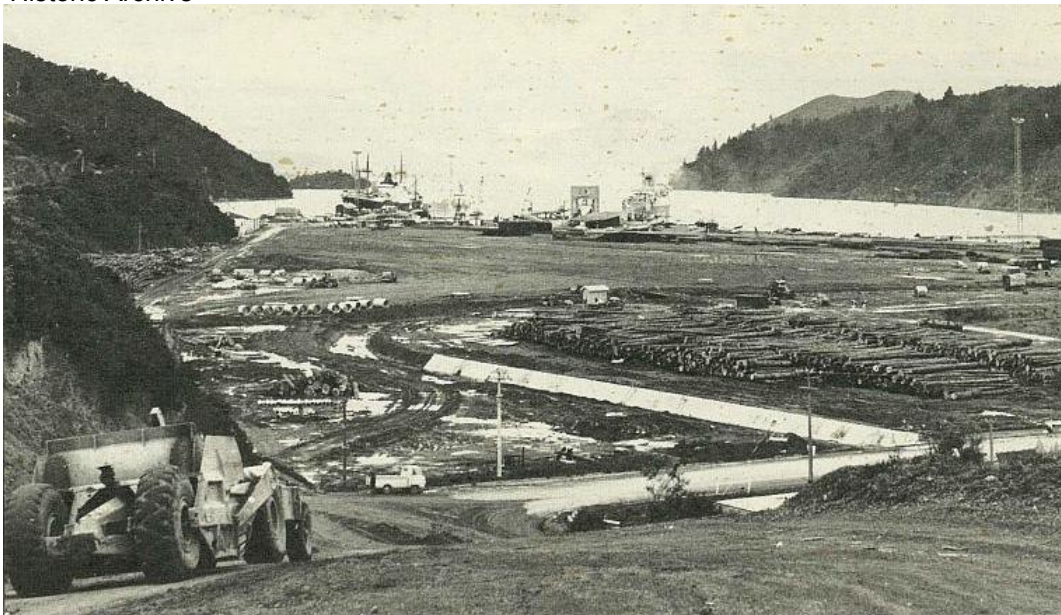
Looking down on to the Picton ferry terminal. At left is the land reclaimed and in the middle of this area a transporter park will be made. The existing terminal, with the Aramoana departing, can be seen near the middle of the photograph. The No.2 terminal will be between that and the Waitohi Wharf alongside which are two ships
