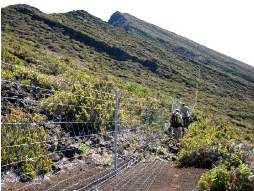
Figure 5: Ungulate-proof fences have been widely deployed in Hawai'i ( above & below ). Note the use of the ground skirt ( below ) as extra protection against feral pigs. (Photos: Maui Now)
