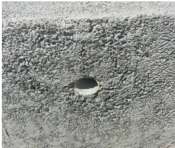
Specific disposal for coral fixing on rocks and habitat for lobster juveniles (Hole)
