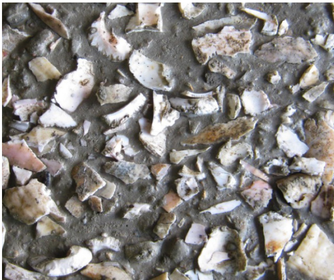
Example of one of the 4 types of eco-designed mooring with specific concrete to enhance coral ecosystem development (Pioch, Sogetras & Ascione)
